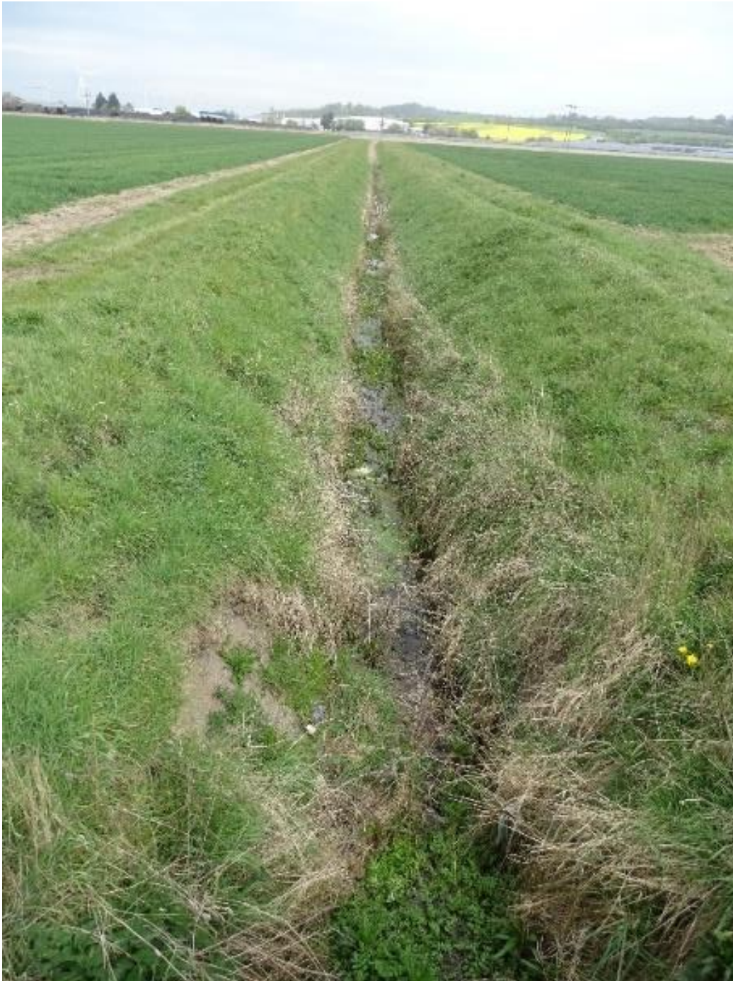
Figure 4-5: Image of ditch to be diverted.
